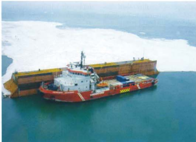
Fig. 5: Ice barrier structure providing shelter for a supply vessel
