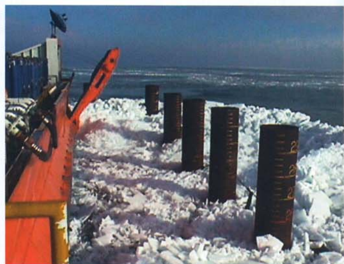
Fig. 2: Ice protection piles, view from drilling unit
