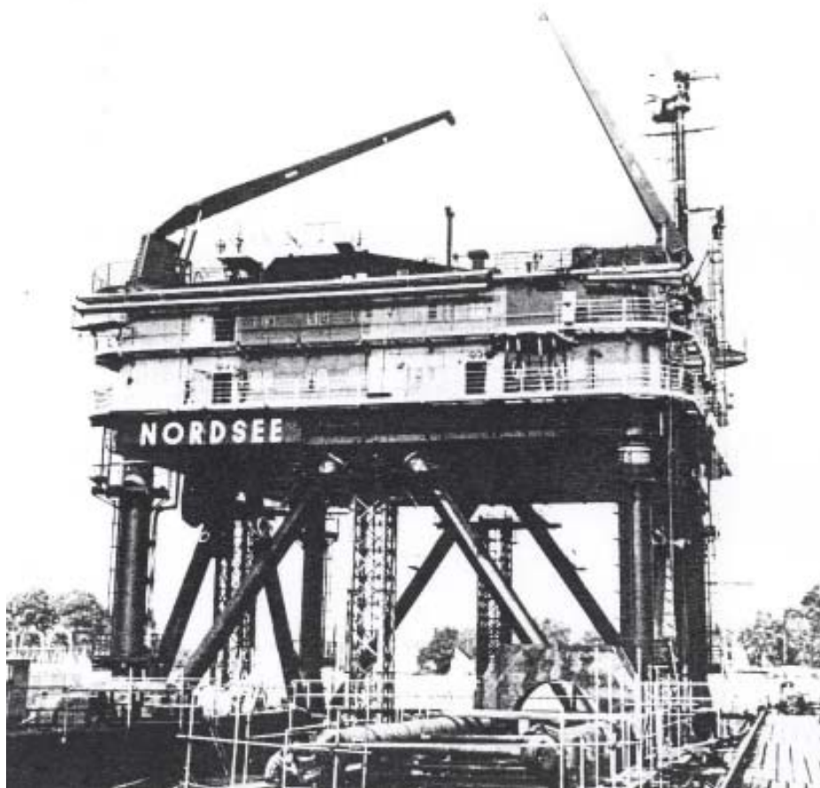
Fig. 7 - Deckhouse and upper tubular structure assembled at the building yard.
