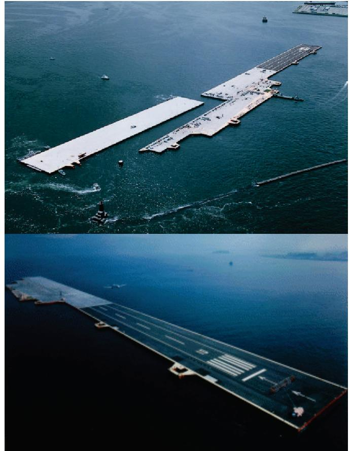
**Figure 3: 1000m Mega-Float floating airport during installation and ready for operation in Tokyo Bay (Ref. [7])**
