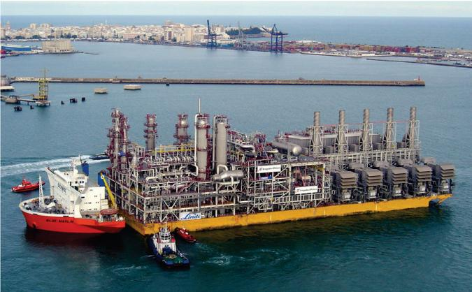
**Figure 4: Float over of the Snøhvit process facility pontoon to the dockship prior shipment to the Arctic (source: Linde)**
